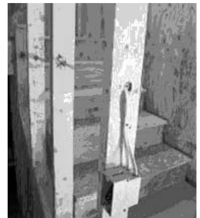
Nonmetallic sheathing helps protect wires from damage.
