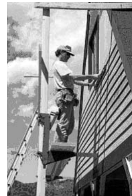
You need to be especially careful when working on scaffolding or ladders.
